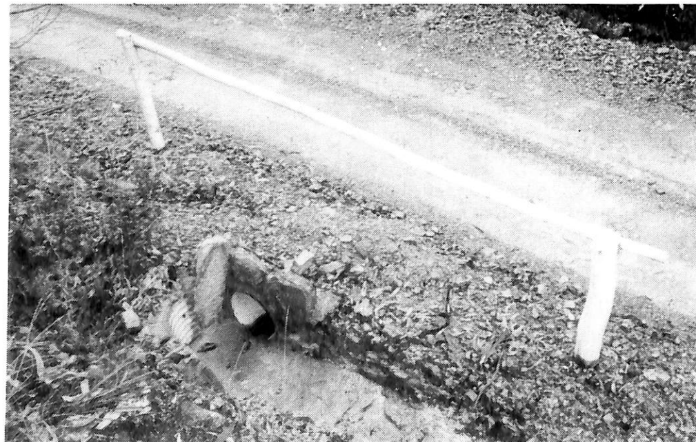
Figure 19 Well constructed culvert with concrete headwall.
