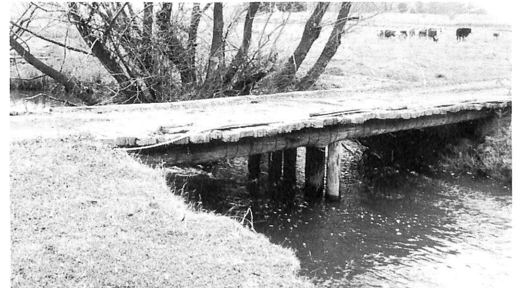
Figure 20 Bridging should cross streams at right angles where possible.
