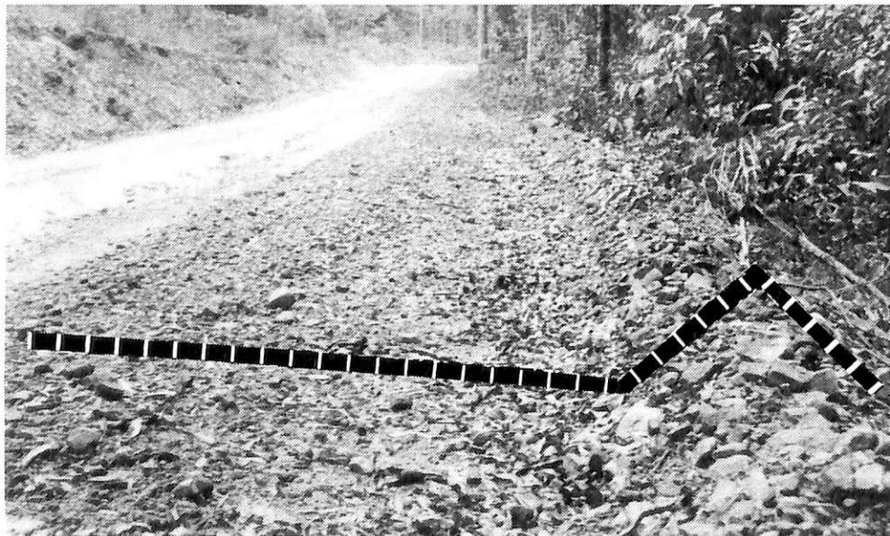
Figure 22 Mounds of earth that build up during construction on the outside of tracks should be removed.
