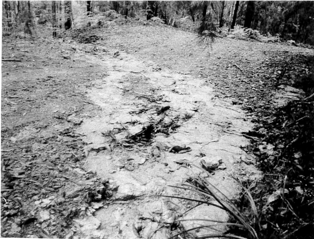
Figure 24 Cross banks should be well compacted with sufficient grade to drain.
