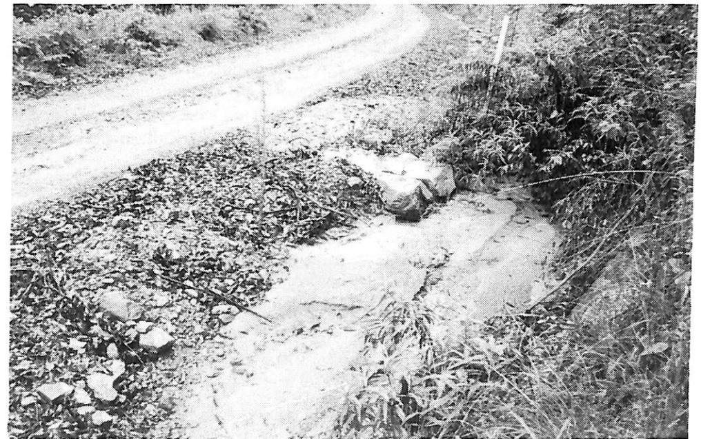
Better siting could have prevented blockage of this culvert.
