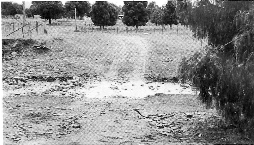
Figure 18 Rockfill ford at natural gully floor level.
