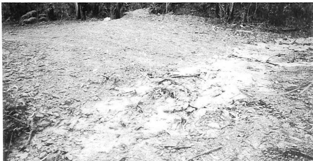
Figure 14 A cross bank directing runoff across the track surface.
