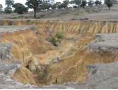
Severe gully erosion.
