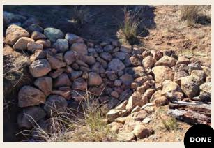
4. Plant, or allow grasses to regenerate below your completed structure. Shrubs may also be planted, though grasses are very effective at slowing water. Any left over topsoil and sod can be placed into gaps in the rocks along with site-appropriate grass seed.
